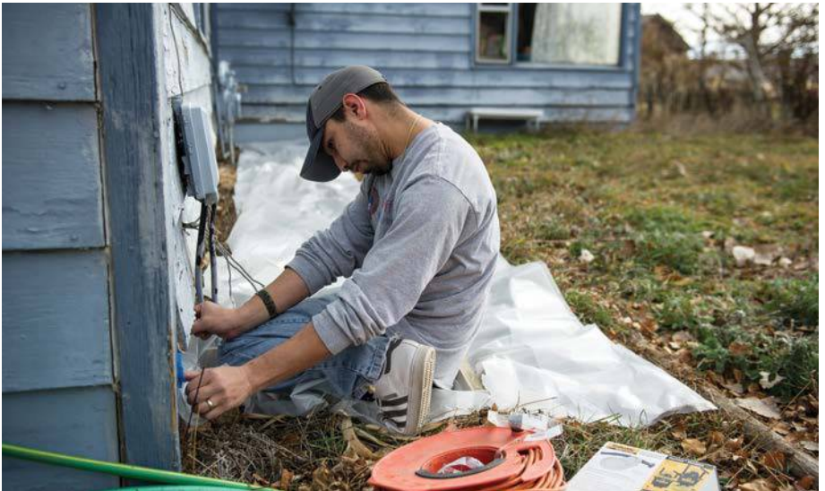
Weatherization can reduce energy bills and improve the efficiency, health, and safety of the home.
