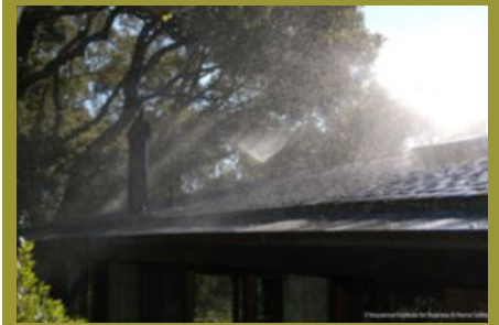
Photo 1. Roof mounted sprinkler.
