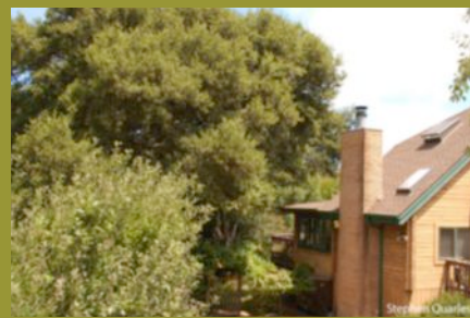
Photo 3. The vulnerability of skylights on a steep-slope roof will depend on the potential for an extended radiant heat exposure to the roof and skylight unit.
