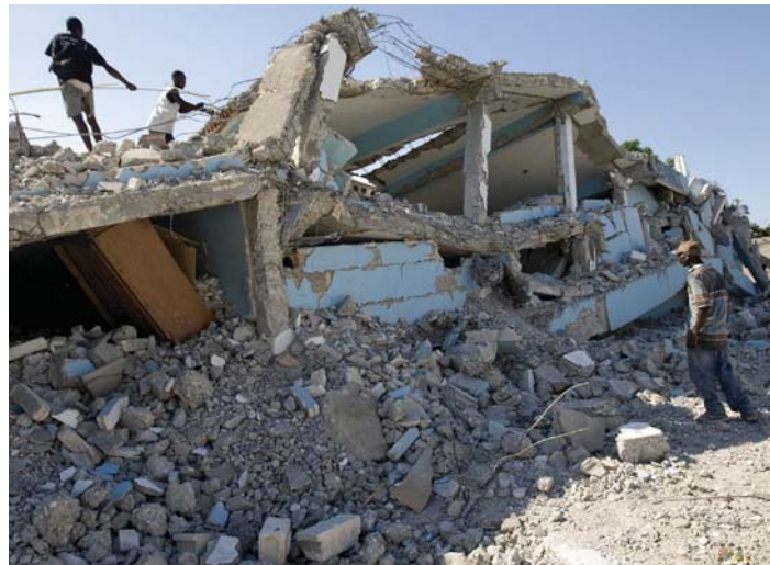
School collapsed by 2010 earthquake in Cité Soleil, Haiti. © UN Photo/Logan Abassi.
