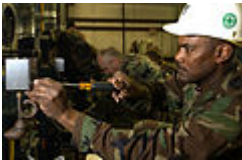
US Navy 030314-N-5862D-088 Utilityman 1st Class Norman Laster, an instructor at Seabee Advanced Utility school at the Naval Construction Training Center sets discrepancies into a heat pack boiler for his students to find during.jpg 3,008 × 1,960; 1.03 MB
