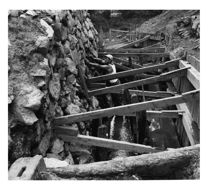
5.6 Robbins working in the tailrace in July 1951. Notice the depth of preservation on the western side of the blast furnace and the upright members of the tailrace. (Photograph 384 by Richard Merrill, 1951.)
