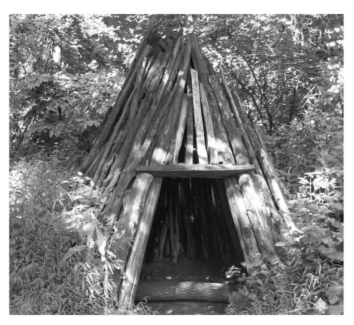
1.7 Reconstructed collier's hut from Hopewell Furnace Na-tional Historic Site. A structure like this would have sheltered the collier when the charcoaling process was underway. (Pho-tograph by William Griswold, 2004.)
