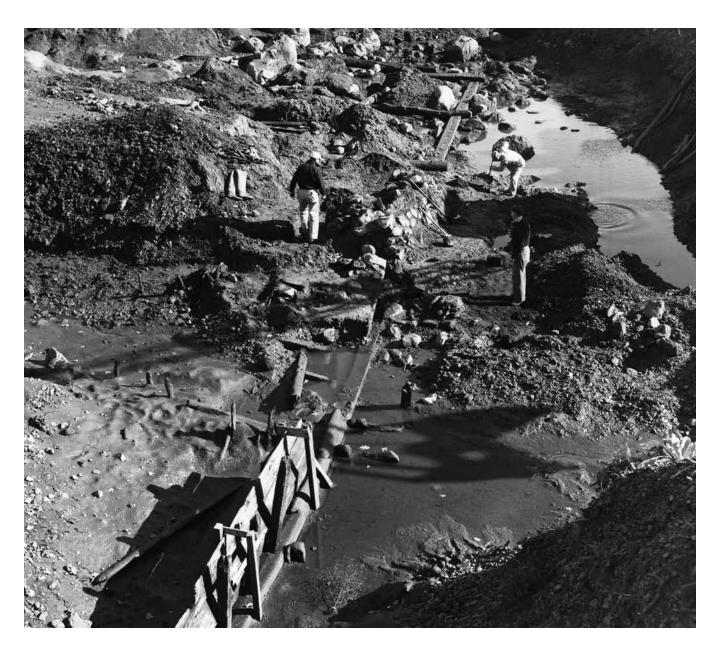
2.12 The bulkhead for the turning basin under excavation. (Photograph 745 by Richard Merrill, 1952.)
