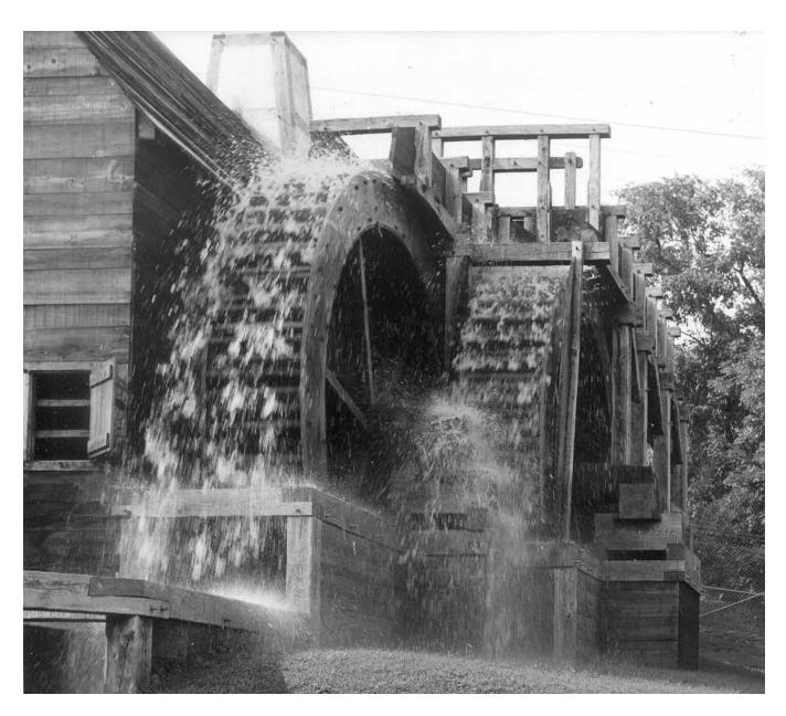
1.4 The reconstructed overshot waterwheels at the Saugus Iron Works slitting mill. (Photograph 1419b by Richard Merrill, 1957.)
