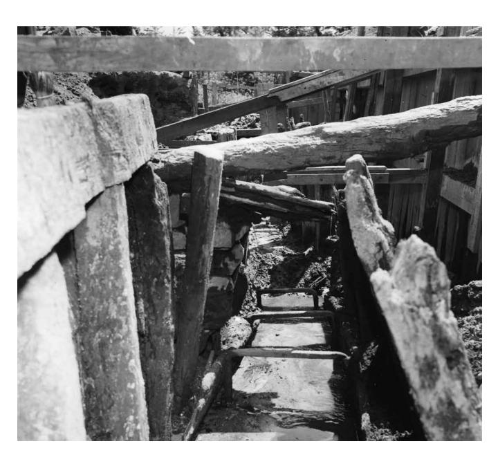
11.2 Close-up view of the blast furnace tailrace with iron staples. (Photograph 411 by Richard Merrill, 1951.)
