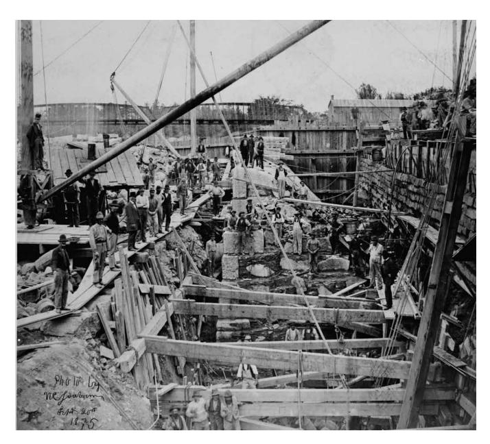
8.2 Dam at the Head of the Pawtucket Falls, Lowell, Massachusetts, September 20, 1875. This photograph illustrates the complexity of dam construction over two centuries after the construction of the dam at Saugus. (Photograph HAER MASS, 9-LOW, 8A-1 from the Library of Congress.)
