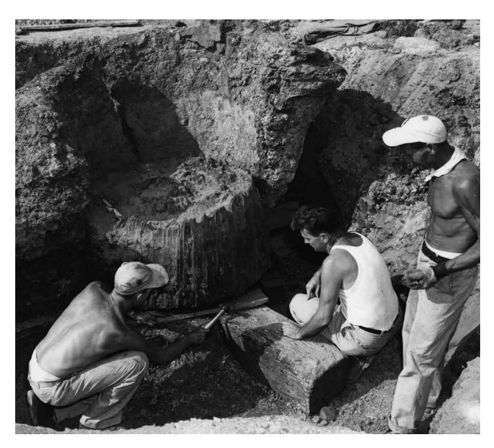
6.10 Removal of the first anvil base block at the refinery forge site. Note shim between block and sills. (Photograph 725 by Richard Merrill, September 1952.)
