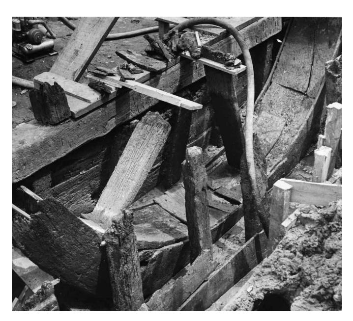
3.12 Intact section of excavated furnace waterwheel, June 13, 1951. (Photograph 362 by Richard Merrill, 1951.)
