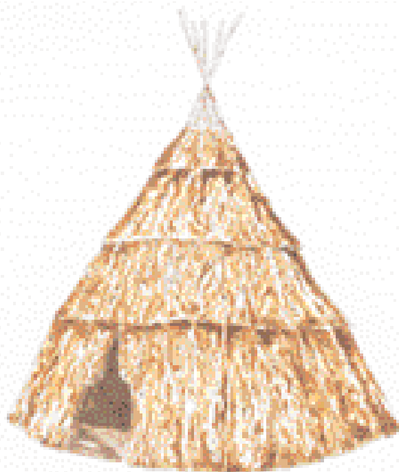
Abenaki conical wigwam with elm-bark covering
